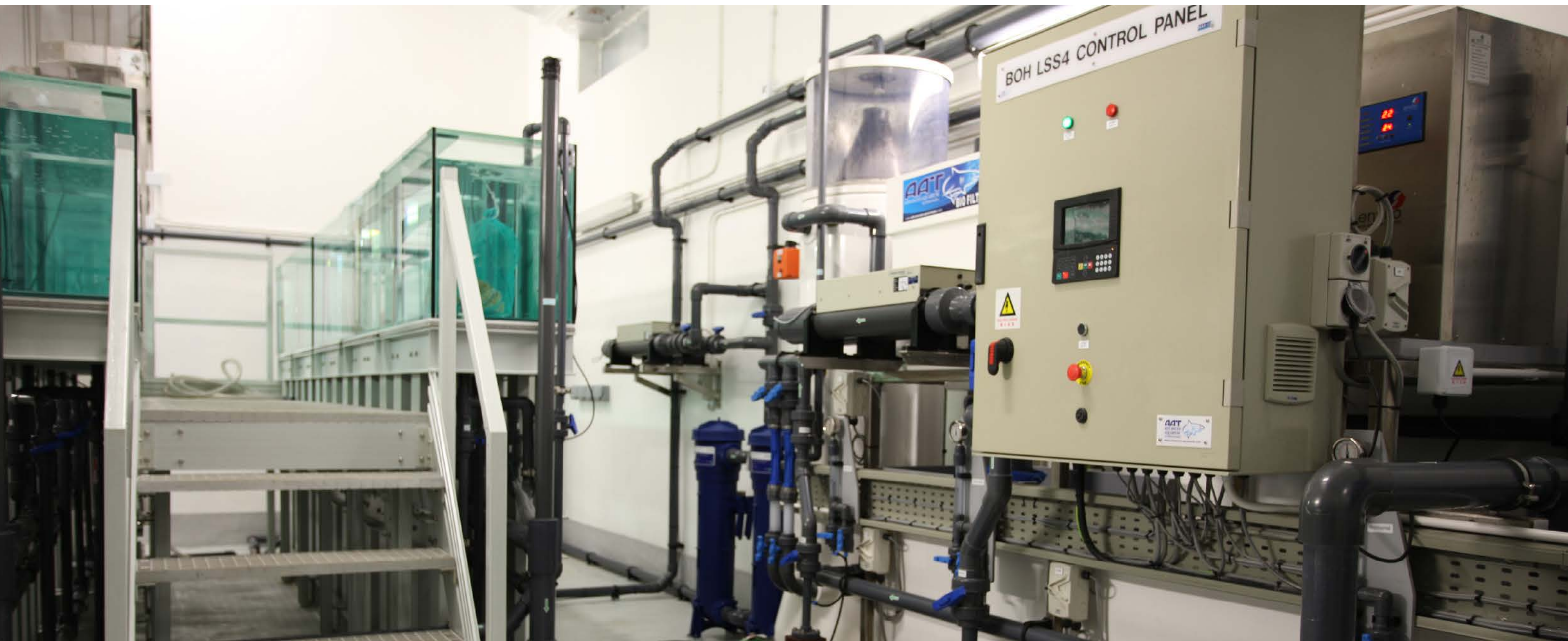
SKID-MOUNTED LSS UNITS
